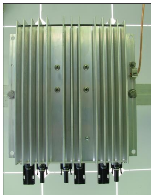
Figure 8: Ampt String Optimizer mounted and grounded
