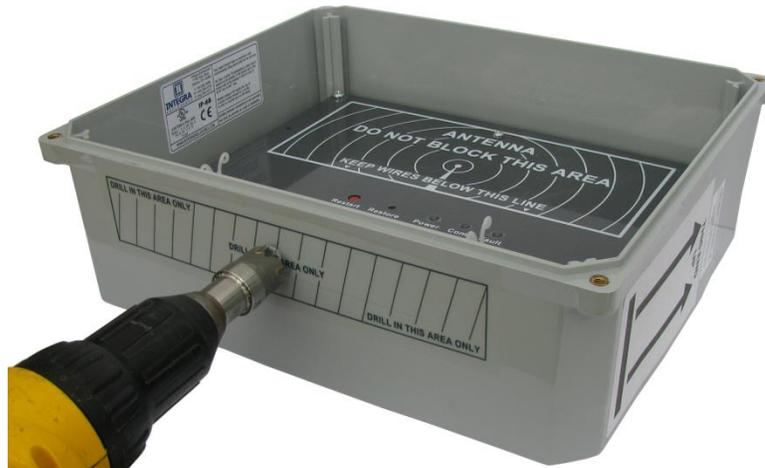
Figure 6: Drill hole for the wire grip within the marked area
