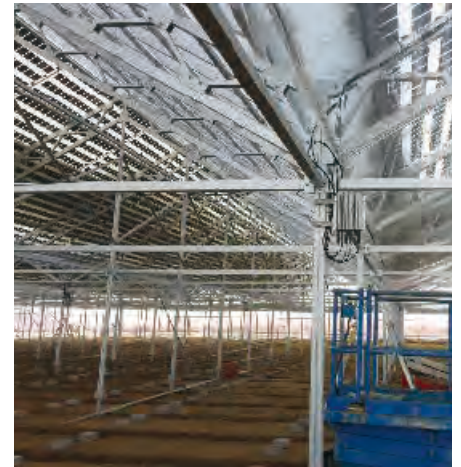
The mega solar power plant has a capacity of 12.7 MW. Tall panels are installed in some areas for a solar sharing project. Crops grow under the panels.
