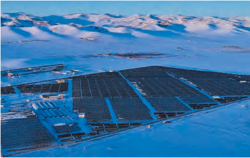
The mega solar power plant has a capacity of 12.7 MW. Tall panels are installed in some areas for a solar sharing project. Crops grow under the panels.
